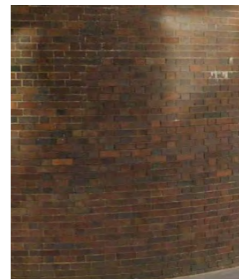
Barbican Stair Tower
