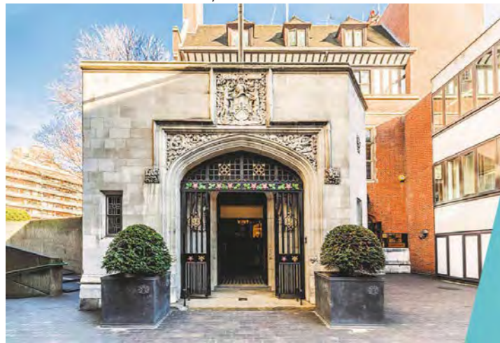
Pointed stone archway at Ironmongers' entry porch
